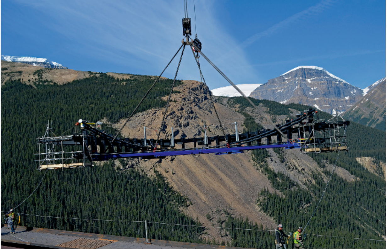
Skywalk module lifted into place.
